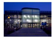
Pilkington Profilit™ is a U shaped profile glass. In standard configurations it is set within a perimeter aluminium frame in singular, double or triple glazed format. The modular nature of the system renders it a flexible design component perfect for inclusion within both exterior and interior projects.
