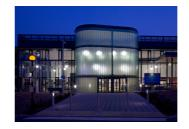
Pilkington Profilit™ is a U shaped profile glass. In standard configurations it is set within a perimeter aluminium frame in singular, double or triple glazed format. The modular nature of the system renders it a flexible design component perfect for inclusion within both exterior and interior projects.
